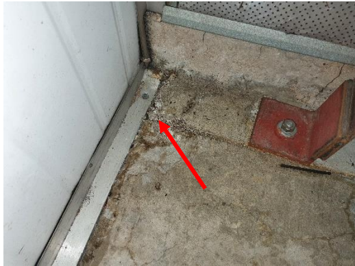
Image 3: Pre-Filter Room - Vermiculite debris
